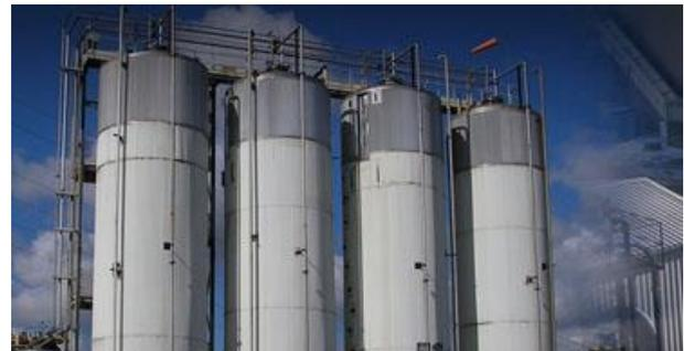
An RFID tag was installed on each tank to uniquely identify each vessel. This now allows inspectors to use a handheld RFID scanner to interrogate the tag.
